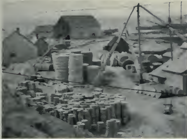
The Grindstone Yard of the Read Stone Co., Stonehaven, N.B.
